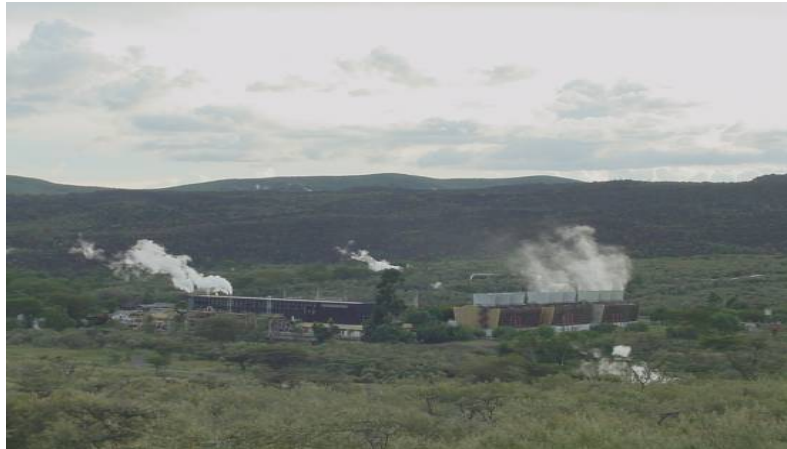
45MWe Olkaria I Power station
