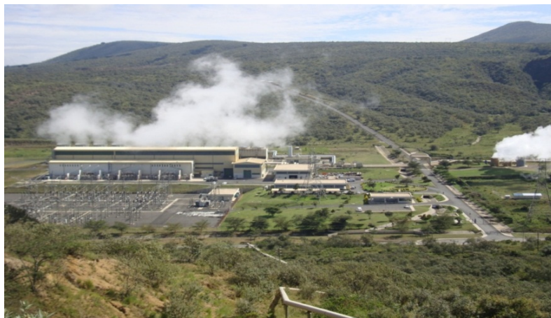
105 MWe Olkaria II Power station
